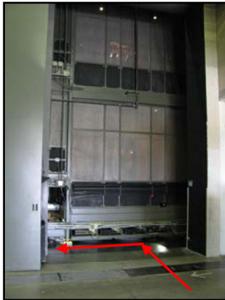
Stage Door w/ Seating Tower Blocking
