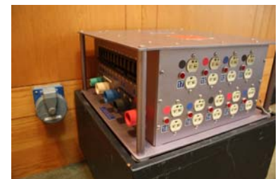
Distro Box w/ Pin & Sleeve plug
