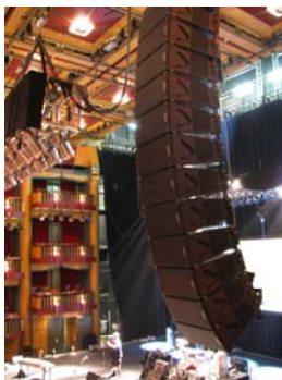
View Showing Arena Line Array
